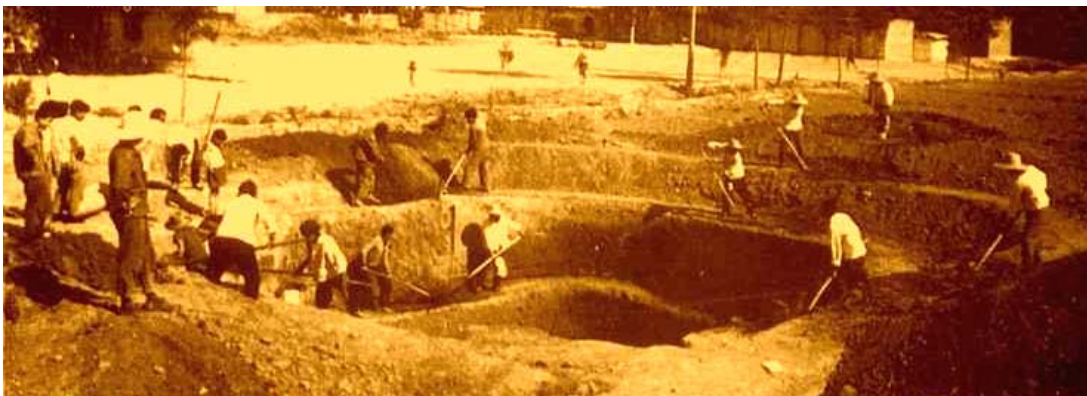
Figure 5 – Excavation of the Fu Hao tomb [15].
