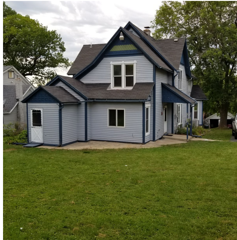
Rear house view from back lawn
